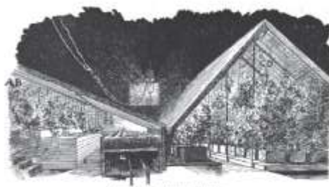
Construction of the electric light house.
